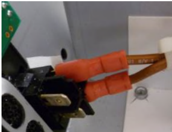
Wiring to mains switch
